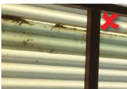
**Over time, conventional sheet lapping is prone to build up of foreign matter and this becomes unsightly.** Regular maintenance of the polycarbonate sheeting surface itself is sufficient to keep the surface clear of any unsightly build up, however unless the sheeting is removed completely, it is virtually impossible to keep the overlaps pristine.
